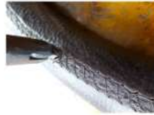
Stitched circular leather handrail.
